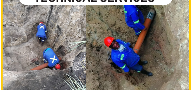
Casting sewer pipeline at Industrial site
