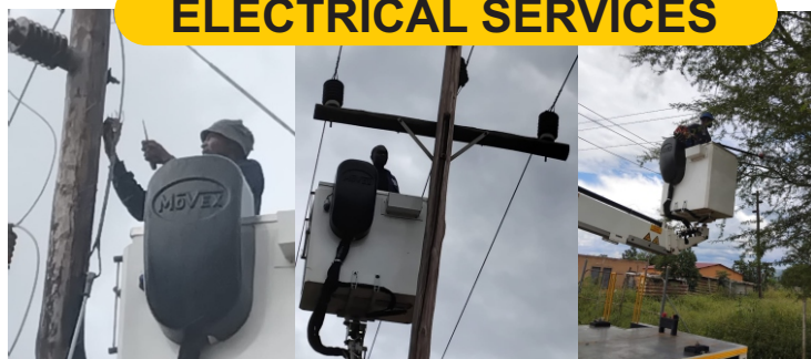
Repairs of loose hanging conductors
