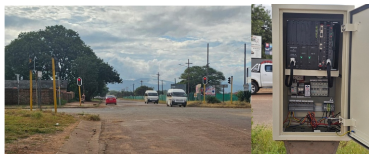
Installation of new traffic signal controller & repair all faulty signals head Cnr Geyser/Dudu Madisha
