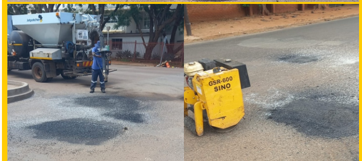
Patching of potholes along Retief Street
