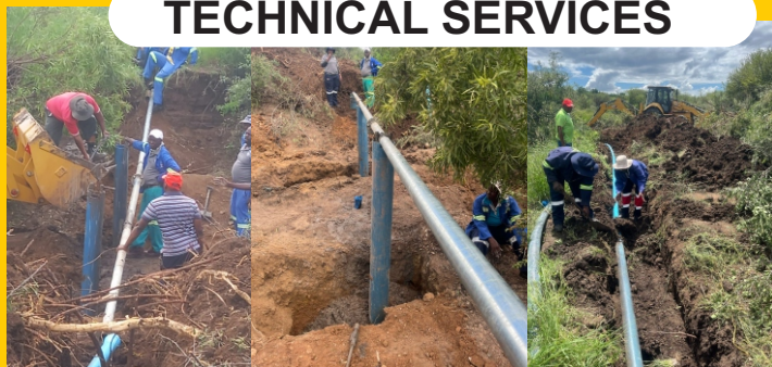
Installaton of the collapsed water pipe line due to recent heavy rainfalls
